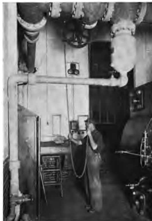
Fig. 2. Valve equipped for Floor Operation.*
